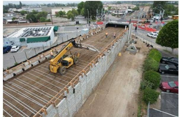
Meanwhile, crews continue to construct the retaining walls for the east approach to the bridge. As seen in the photo above (right), the retaining walls for the approach now have been built all the way to the east abutment. When completed, the east approach will measure nearly 1,300 feet in length.
