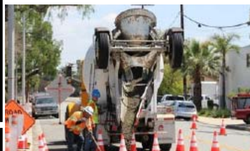
Gold Line Utility Relocation Work Underway
