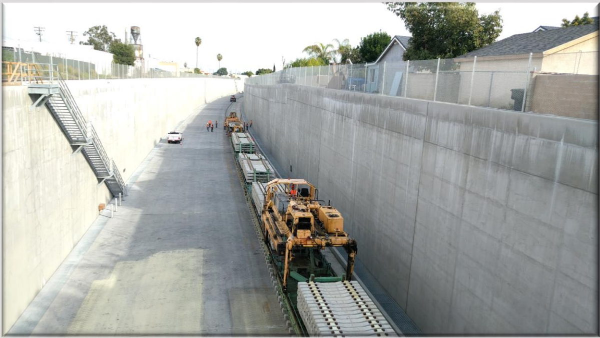
LAYING TRAIN TRACK – SAN GABRIEL TRENCH PROJECT – CITY OF SAN GABRIEL
