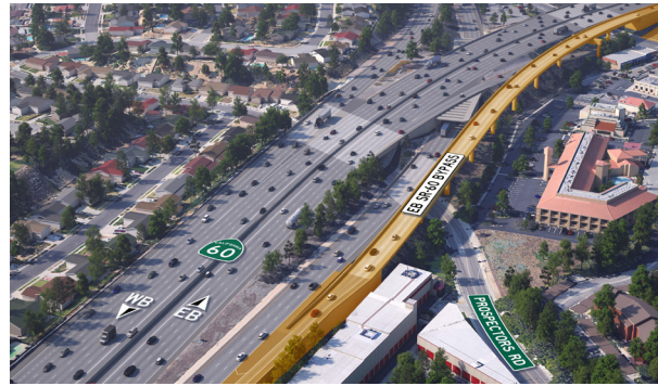
New eastbound SR-60 bypass bridge over Prospectors Road to be used as a new lane on eastbound SR-60.
