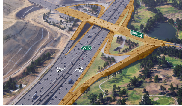
New Grand Avenue bridge with reconfigured on- and off-ramps.
