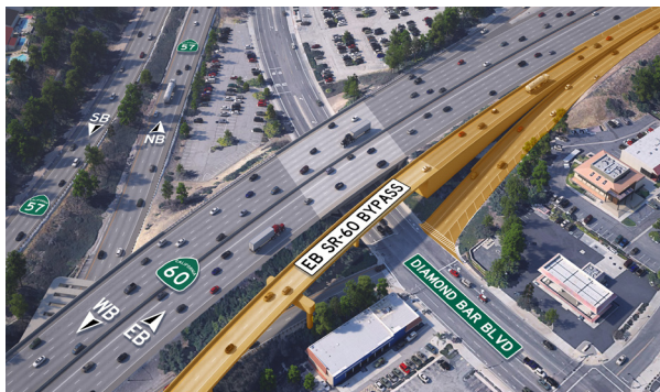
New eastbound SR-60 bypass bridge over Diamond Bar Boulevard to be used as a bypass for eastbound SR-60 commuters.
