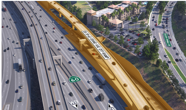
New eastbound SR-60 Grand Avenue bypass bridge exclusively for eastbound SR-60 commuters exiting Grand Avenue.
