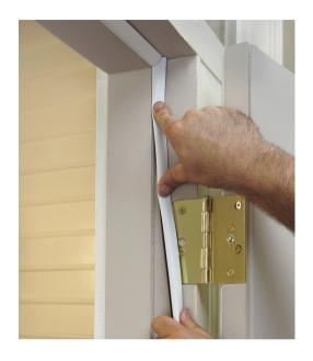
Weatherstripping is a rubber that is used to seal the edges of doors or windows against any air leaving or entering the home. There are various types of weatherstripping as well as different widths and depths. Many come in a self-adhesive form that is easy to install.
