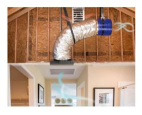
Typically a whole house fan is installed inside the attic, the space between the ceiling and living space. . It works by pulling the cool fresh air from the outside into your home up into your attic and expels hot stale air out the attic vents. The purpose is to extract the heat from the entire home and help the home stay cool longer and requires less usage of the AC unit.
