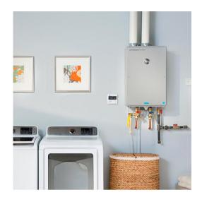
Tankless water heaters provide hot water only as it is needed, compared to standard water heaters that store hot water in a tank where it could lose heat and waste energy.
