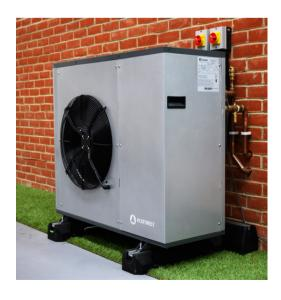
A heat pump is an energy-efficient alternative to furnaces and air conditioners. They use electricity to transfer heat from a cool space to a warm space, making the cool space cooler and the warm space warmer. The most common type of heat pump is the air-source heat pump, which transfers heat between your house and the outside air.
