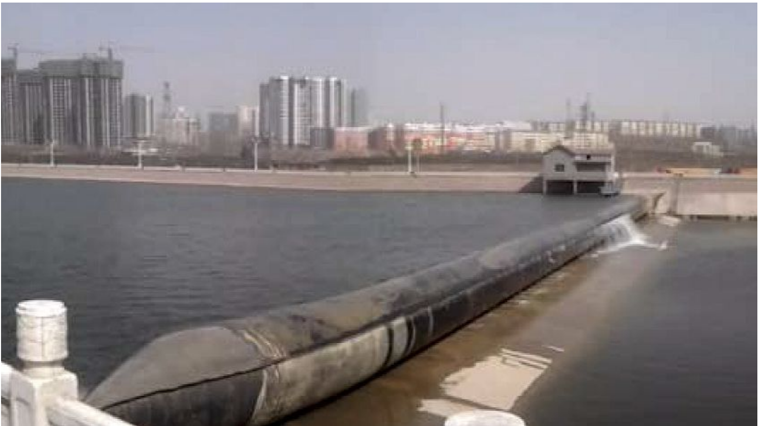
A prototype of an inflatable dam. Los Angeles Bureau of Sanitation
