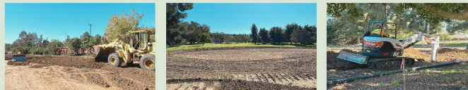
Grading new fairways #1 green under reconstruction New irrigation pipe installed
