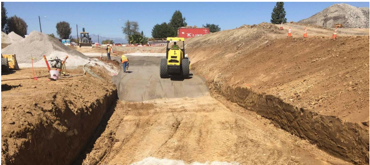
Fullerton Road (Retaining Wall Excavation)
